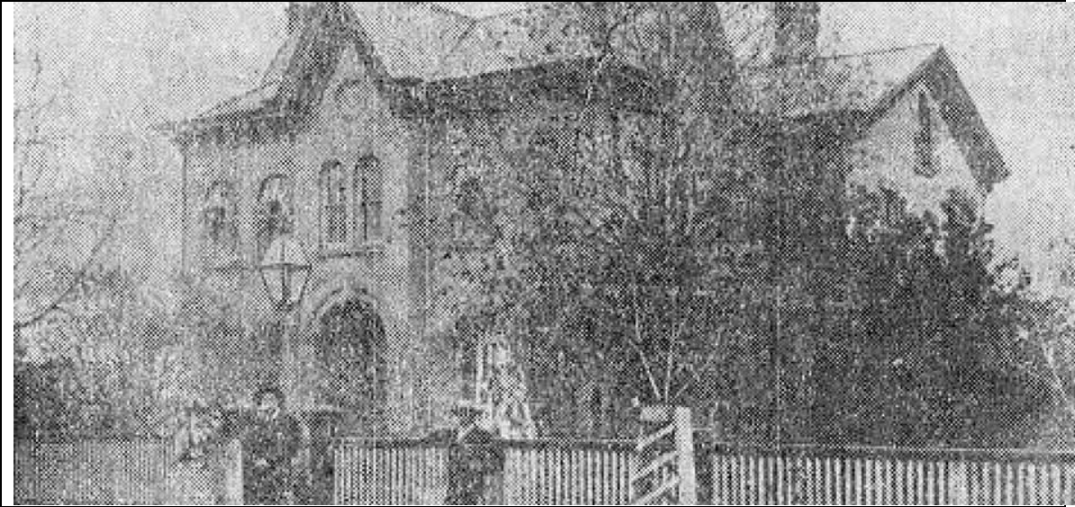
Site of the Whitney-Trott House1 Main Street across from Chilton Avenue Built 1861
